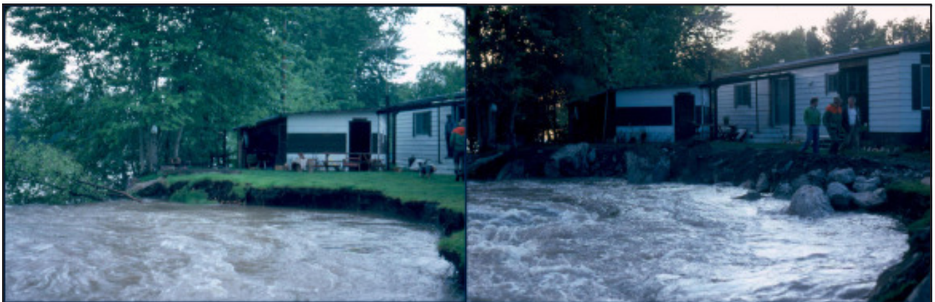
This house on the West Gallatin is seen during a flood. With the river shifting towards the house, emergency riprap was installed to protect the home. Bank stabilization is virtually always authorized after a home is built. Photo by Gillilan Associates, Inc. of Bozeman.
