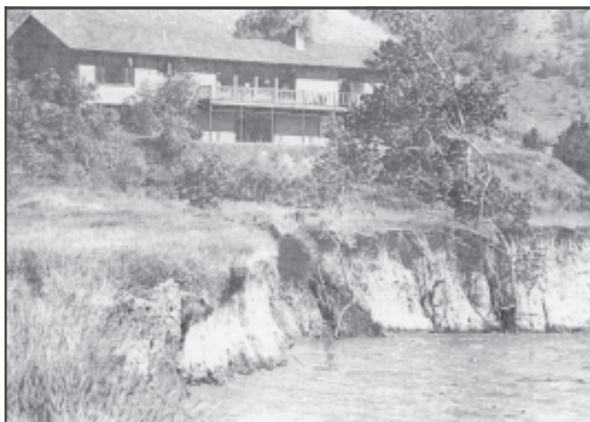
This home on the Yellowstone River in Park County did not need a floodplain permit. On the left, the house is shown in 1996. On the right, the same house is shown after the 1996-97 100-year floods, just before it was destroyed. Many of Montana's streams and rivers located in valley bottoms meander. A flood can shift the main stem of the stream or river hundreds of feet. Both photos are from the DNRC photo library.
