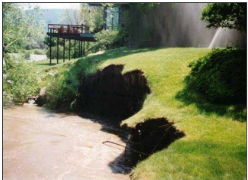
Lawns do not filter out pollutants. With native vegetation, water flows through the vegetation. With lawns, water flows over the surface. Montana Dept. of Natural Resource and Conservation (DNRC) photo library.
